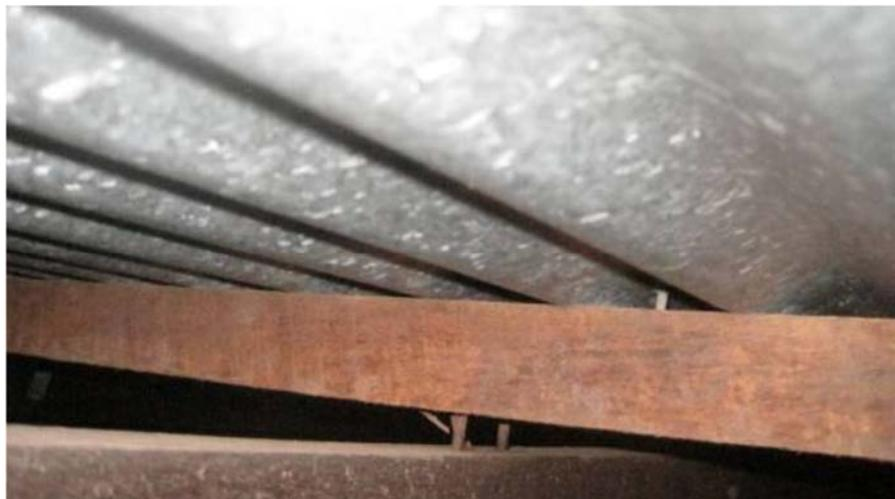
*Figure 2.4 Hidden damage of batten to rafter connections caused by TC Yasi (Boughton et al. 2011)*
