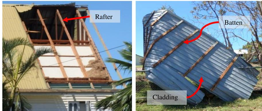
Figure 1.1 Typical batten-rafter connection failure: a large section of the roof envelope removed (right) with cladding still attached to battens and rafters left intact (left). Adapted from Boughton et al. (2017)
