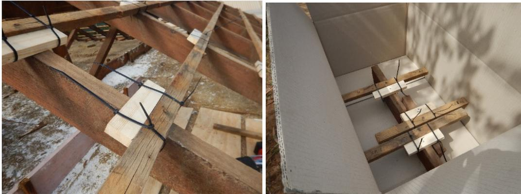
Figure A.2 Connections being prepared for extraction (left) and being packed for transit (right).
