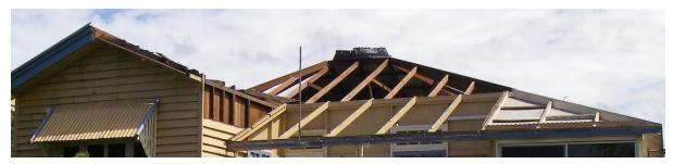
Figure 2. Part of the roof cladding with battens still attached flipped on to the leeward side
