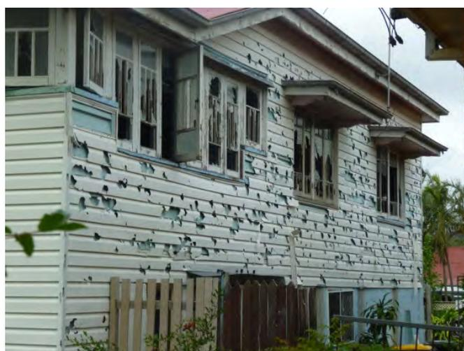
**Figure 7:** Hail damage to windows and vinyl cladding of an older house. The proximity of the neighbouring house on the right and the size of the window shades suggest hail being driven at a sharp angle by the wind.
