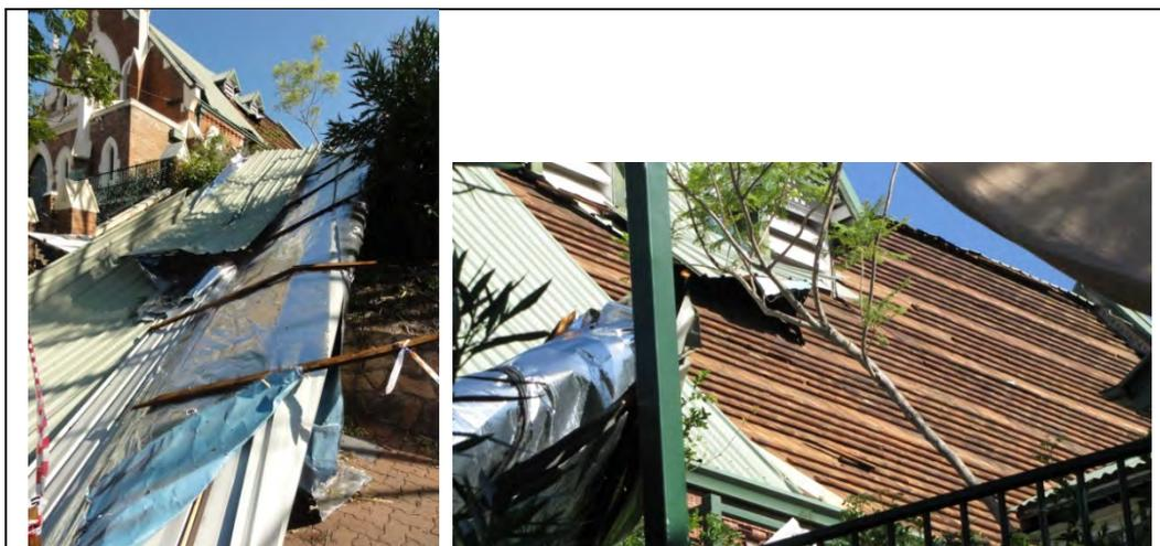
**Figure 3:** Loss of metal cladding and battens of a church. Originally a tile roof, the new metal roof was only secured to every 6<sup>th</sup> timber batten.
