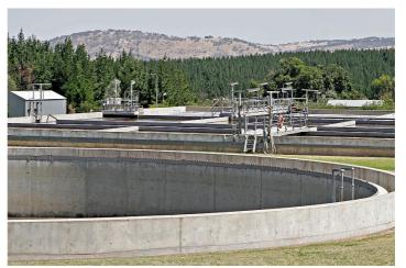
environmentally safe treated wastewater. A by-product of waste water treatment is usually a semi-solid waste or slurry called sewage sludge that has to undergo further treatment before being suitable for disposal or land ,,,,,,,,,,,,,,,,,,,,,,,,,,,,,,,,,
