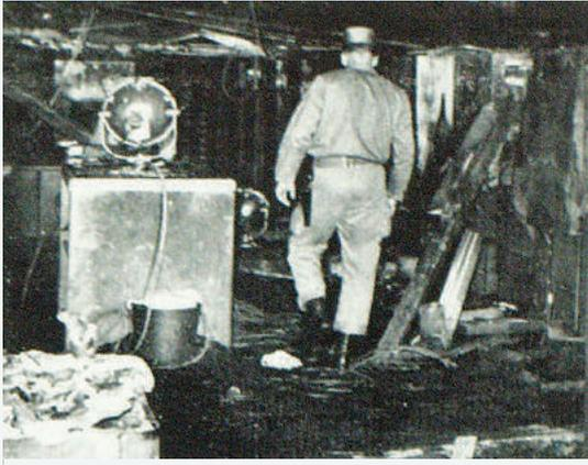
Started by a temporary light bulb igniting a fibreboard ceiling, the fire went on to burn an area of 370 m<sup>2</sup>.
