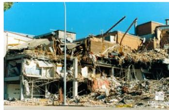
Figure 1. Damage to reinforced concrete frame building following the 1989 Newcastle Earthquake.
