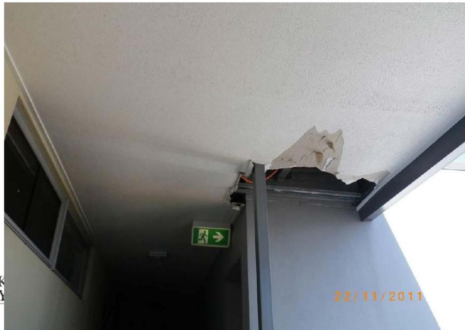
Inadequate box gutters for roof area.
