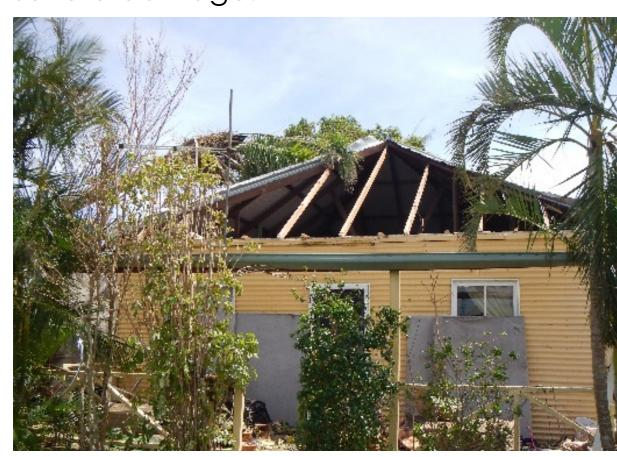
There were cases of older housing with relatively new roof cladding installed to contemporary standards (i.e. screwed fixing as opposed to nailed) but lacking upgrades to batten/rafter or rafter/topplate connections, loosing roof cladding with battens attached.
