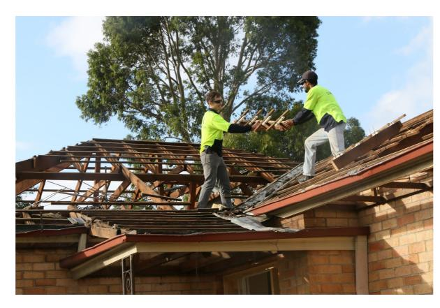
The primary structural components of a pitched roof frame include the rater to wall, ceiling joist to rafter, collar tie and rafter to ridge beam connections.
