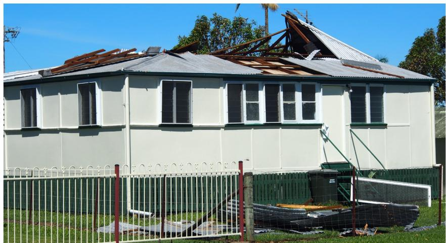
Figure 1: Severe structural roofing failure in Proserpine from Tropical Cyclone Debbie.
